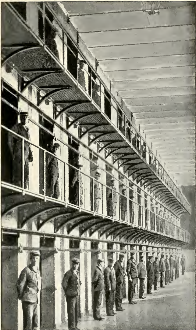
Section of Cell House A, Huntingdon Reformatory.
